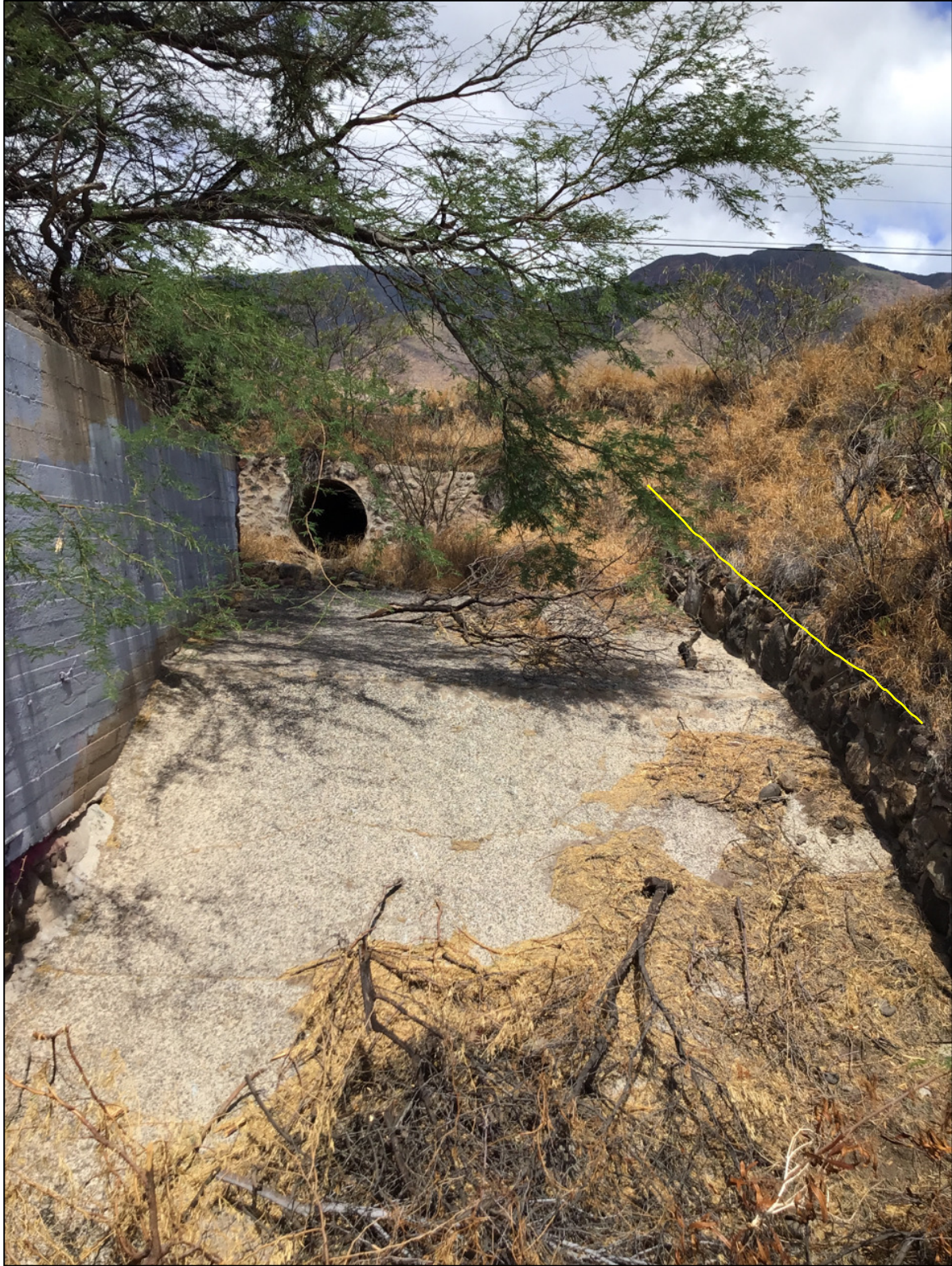
Photo 23. Awalua Stream concrete culvert (east view) location of transect between the inner (unnamed) paved road and the Honoapiilani Highway. The south side rock wall feature (yellow line) with the vegetated bank was used to determine the OHWM level here.
