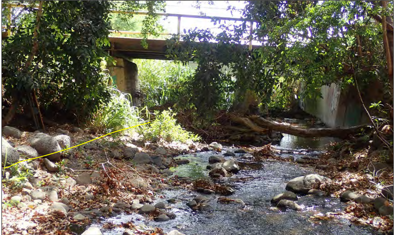
Photo 86. Location of Transect 3 At the Olowalu Stream Bridge; Sediment Staining on the Concrete Bridge Contributed to Determining the OHWM Level in this Area
