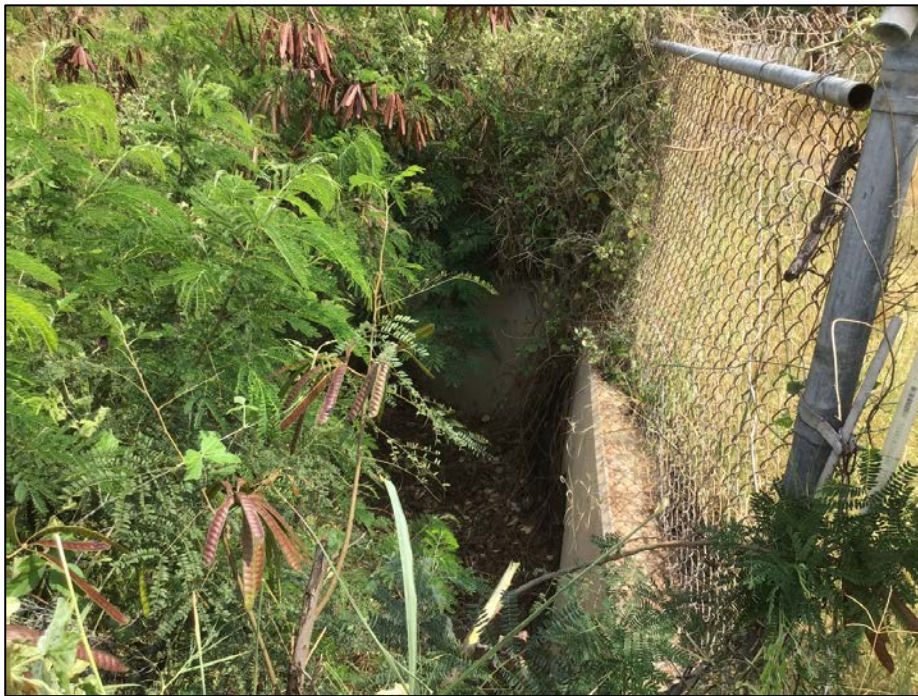
Photo 17. Ekehene Street culvert (south opening on top and north opening below) was overgrown with vegetation at the time of the 2025 survey.
