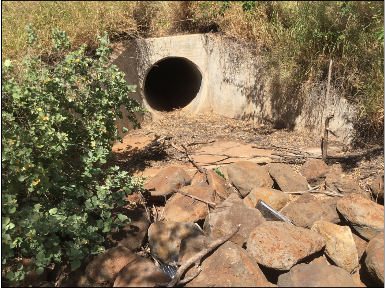
Photo 25. The top beam and the wings of the concrete culvert were used to delineate the OHWM level at this feature.
