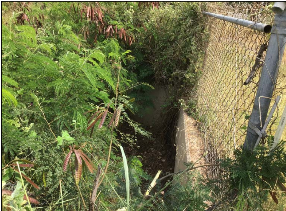
Photo 14. Ehehene Street culvert (south opening on top and north opening below) was overgrown with vegetation at the time of the 2025 survey.
