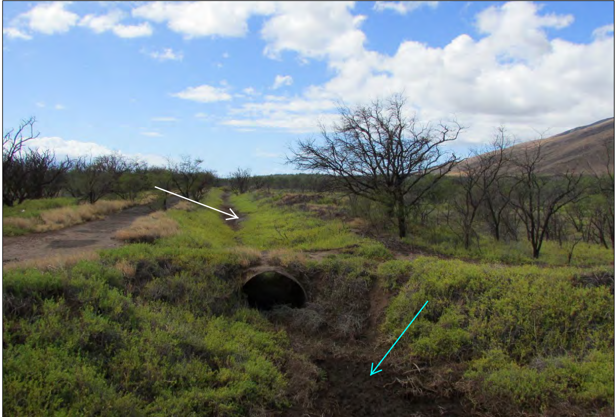
Photo 63. Culvert Connecting the North-South Ditch 7 (White Arrow) to the Hanaula Gulch (Blue Arrow)
