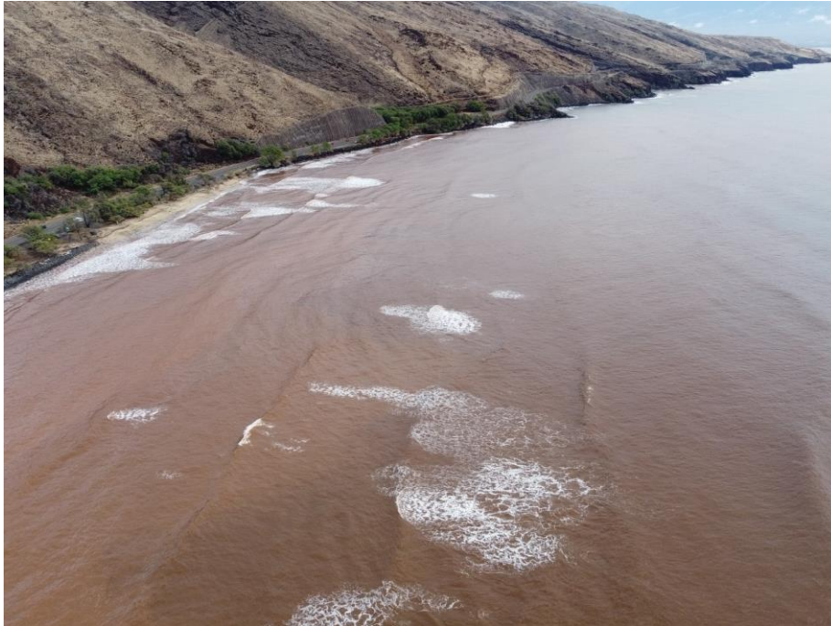
Coastal waters adjacent to Pāpalaua retention basin affected by the overflow of the basin during a 2-year storm event. Photo Credit: Jon Brito
